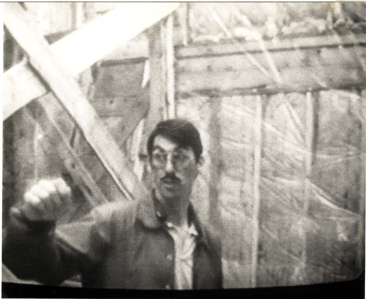
Jerry Oliver shows the new studio under construction at La Grand'Terre.
